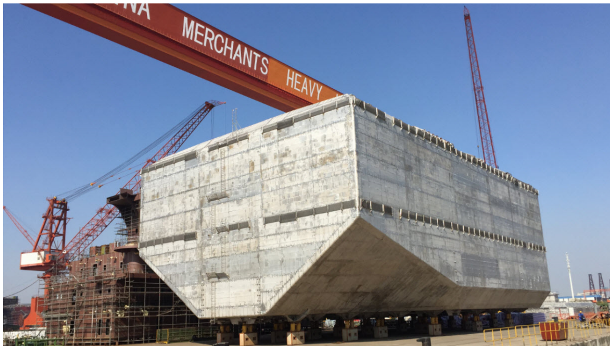
A pre-fabricated tank ready to be lowered into the hold of Saga Dawn (source: LNT Marine)
